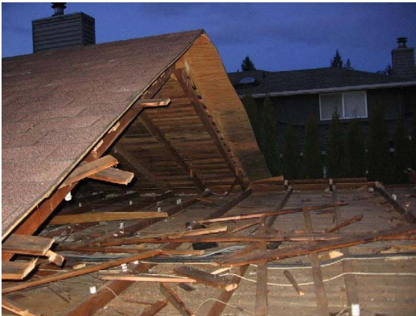
**TAKING OFF THE ROOF:** Now the 'heavy lifting' really gets going, as the crew takes apart the roof, ceiling, and walls.
